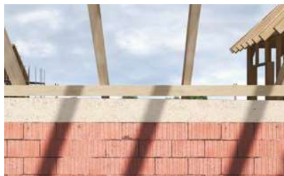
Wooden beams adjustment
